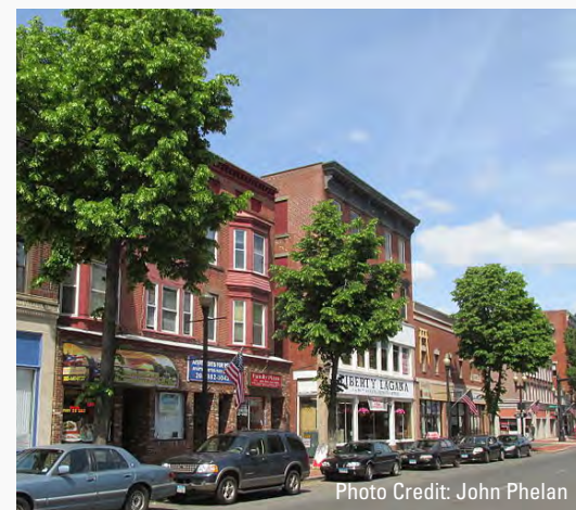
Reconstructed West Main Street sidewalks from Cook Avenue to South Grove Street. Photo Credit: John Phelan
