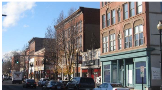
Figure 213-1. Buildings fronting the north side of West Main Street
