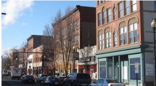
Figure 213-23. Buildings Fronting the North Side of West Main Street
