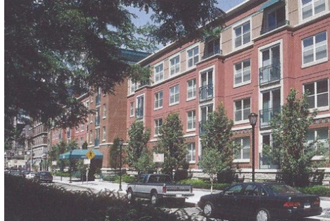
Figure 213-3. Residential building similar to what might be found in the Hanover Sub-District
