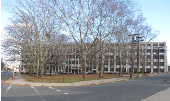
Figure 213-2. A pocket park along Pratt Street in the Park Sub-District
