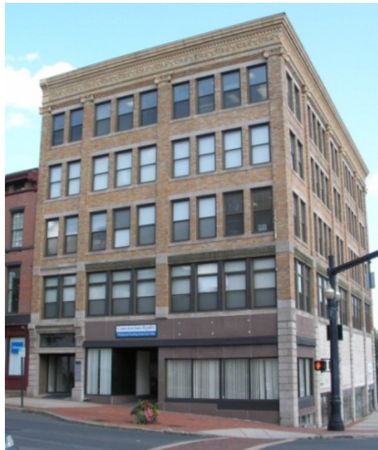
Figure 213-22. Hall & Lewis Building [1910]
