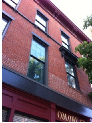
Figure 213-19. Traditional Materials and Punched Openings in the Historic-Commercial Sub-District
