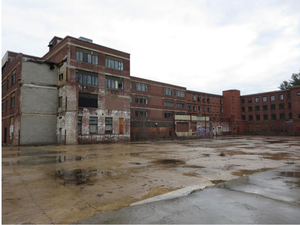
Photo 1: East Elevation of 116 Cook Ave. Building Complex
