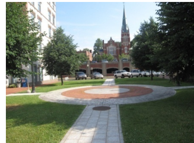
VIEW OF CORRIDOR TO THE NORTH TOWARDS PLAZA
