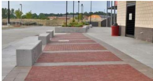
Sidewalk paver/concrete banding
