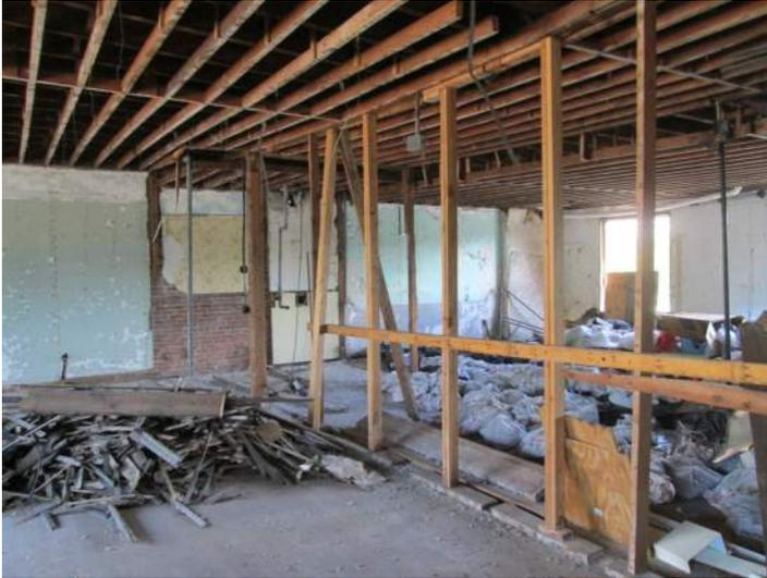
*Third floor framing showing removed bearing wall and shoring repairs..*
