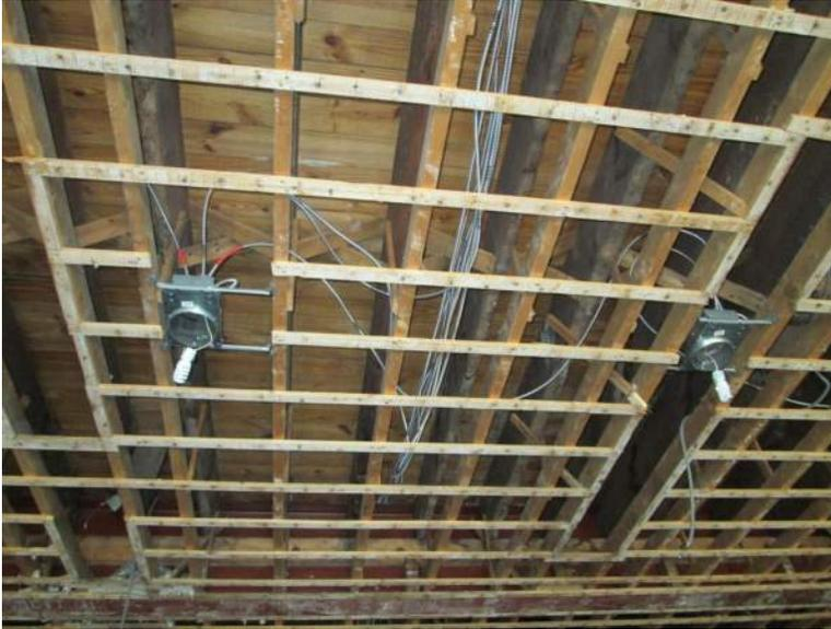
*Third floor framing showing original framing members, repaired subfloor above, and secondary ceiling framing with some new electrical rough-ins.*
