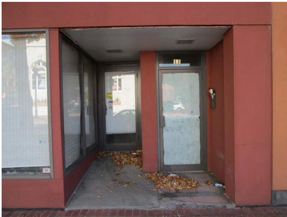
*Front façade improvements consist of stucco application on the existing building. The storefront construction is near the end of its useful life.*
