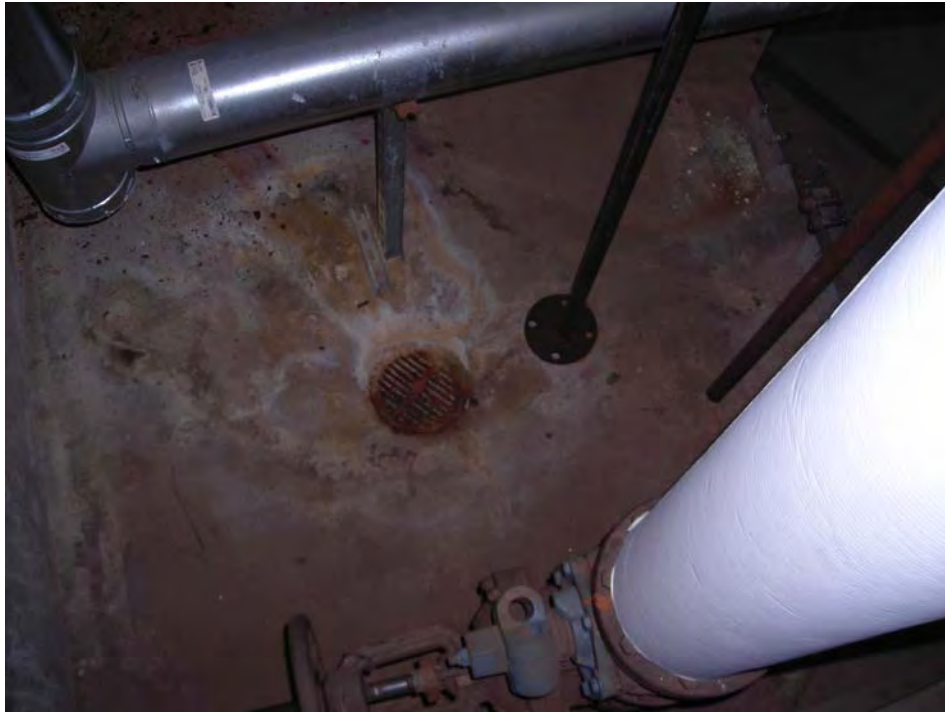
Photograph 3 – Floor drain in boiler room. New gas-fired boiler is to the right of the drain.
