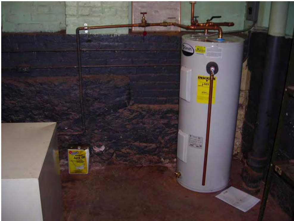
Photograph 10 – Electric hot water heater and 1-gallon can of hydraulic jack oil on ground floor of building.
