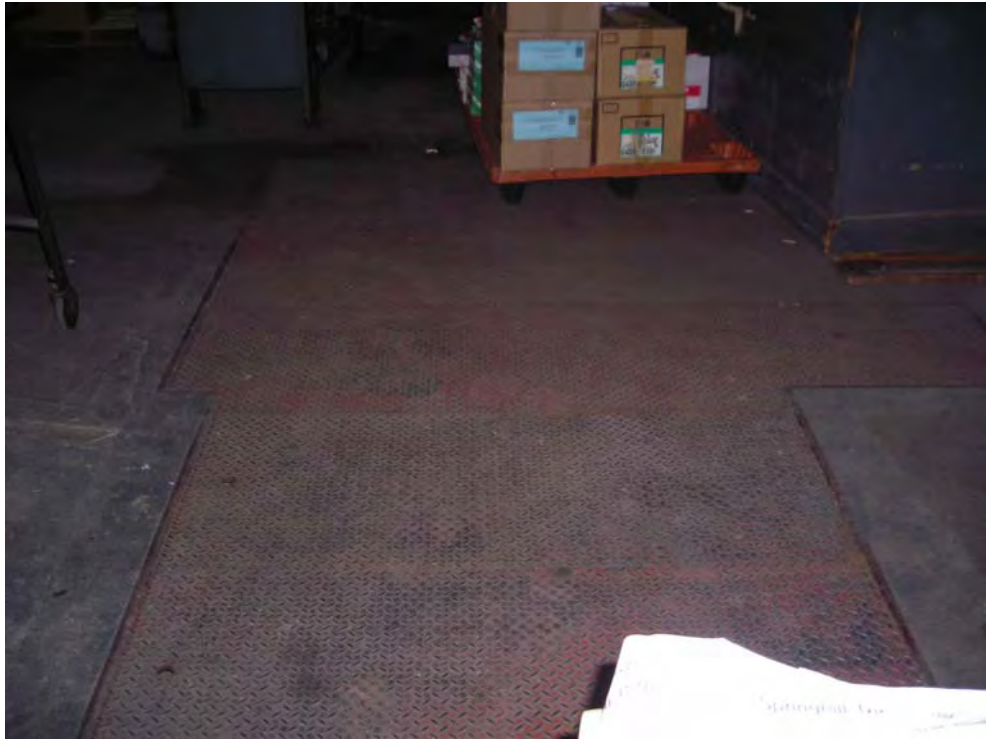
Photograph 9 – Large steel plates in former circulator printing shop on ground floor.
