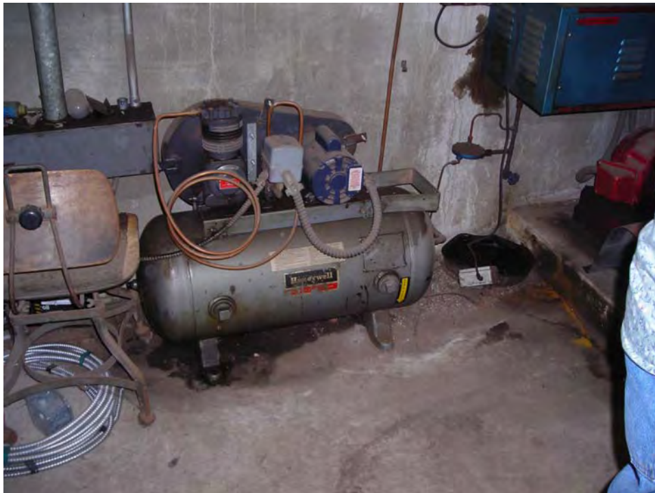
Photograph 4 – Air compressors in boiler room that are leaking oil on floor and wall. Drip pan full of oil is on the floor to the right of the silver compressor and underneath the blue compressor.
