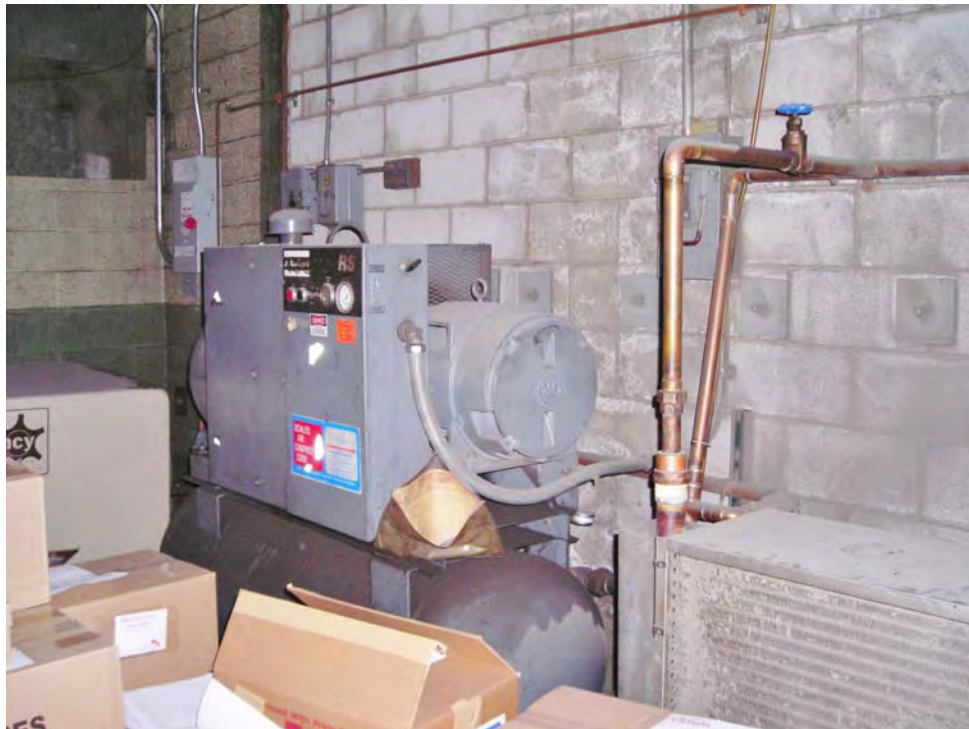
Photograph 19 – Compressor coated in oil in southeastern portion of former paper storage room.
