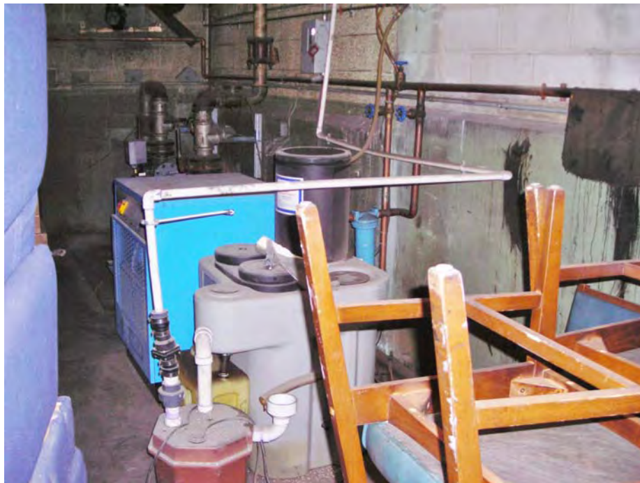
Photograph 18 – Oil water separator and compressor in southeastern portion of former paper storage room.
