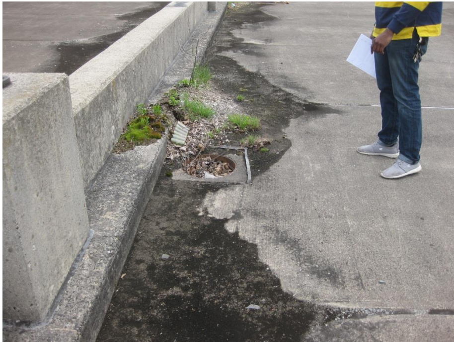
Photo K-5 – Clogged Roof Drains
