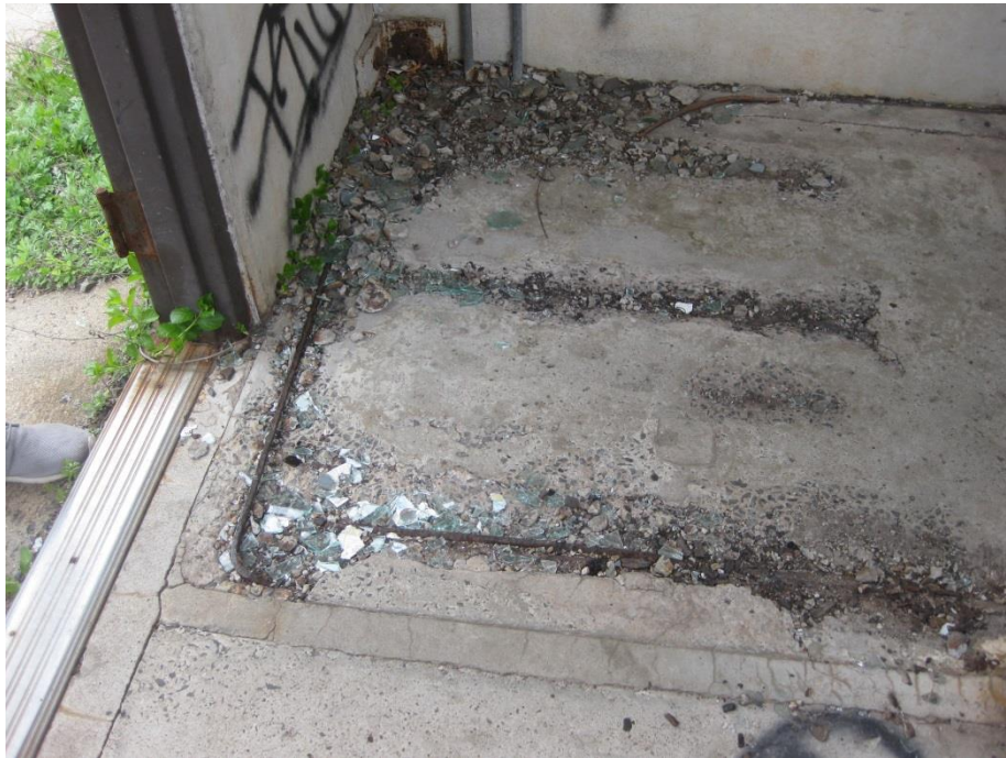
Photo K-3 – Damaged Concrete at Stair Platform
