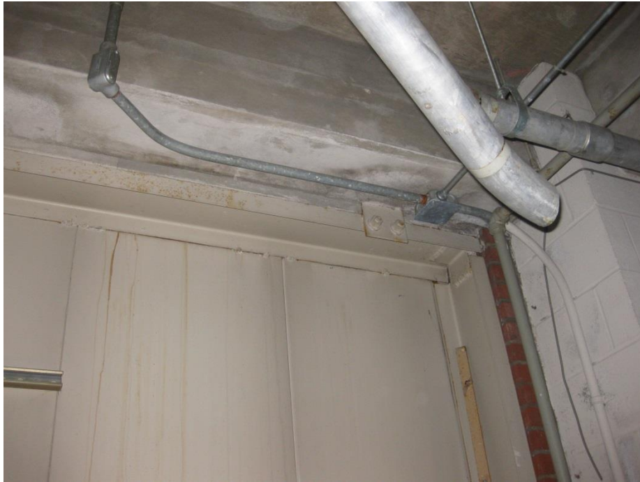
Photo D-1 – Water Infiltration at Penthouse at 1952 Addition
