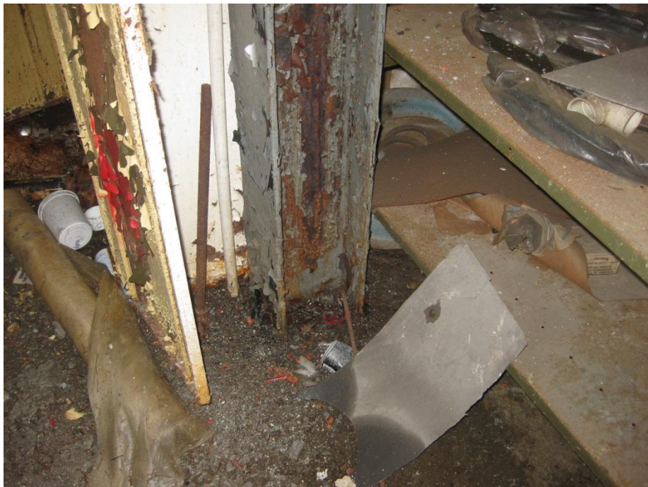
Photo I-3 – Corrosion at Steel Columns and Baseplates
