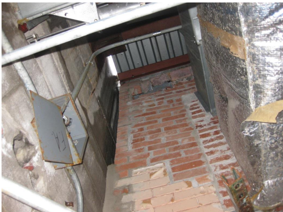
Photo I-1 – Water Infiltration at Expansion Joint
