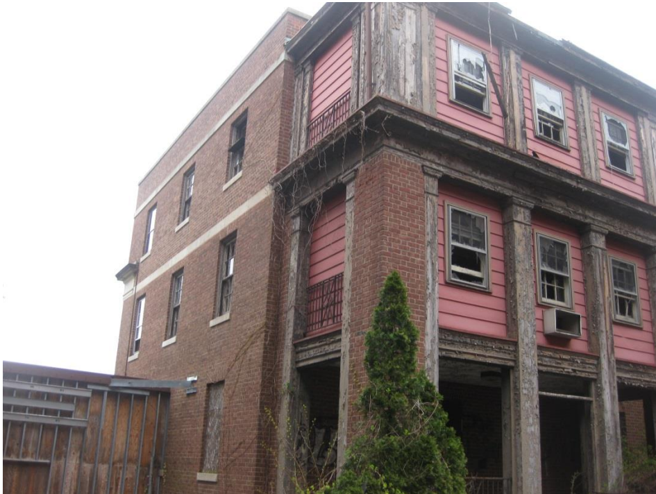
Photo A-2 – Damaged Wood Structure at Nurses Home
