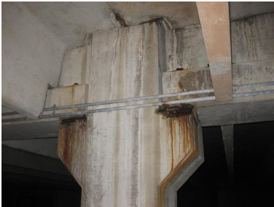
Photo K-6 – Rust at Bearing Plates
