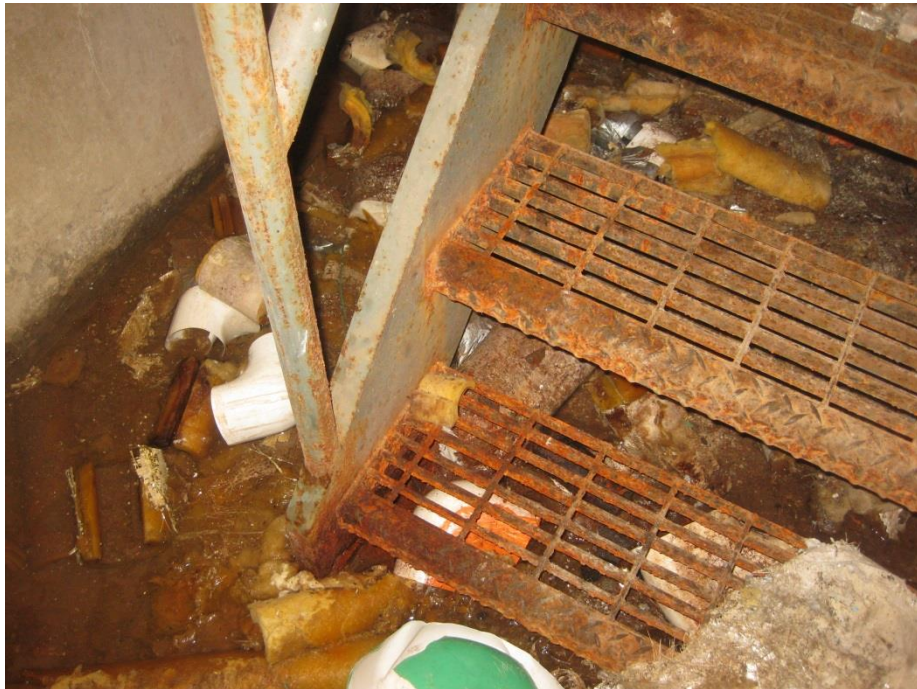
Photo I-10 – Damaged Stairs at Boiler Room
