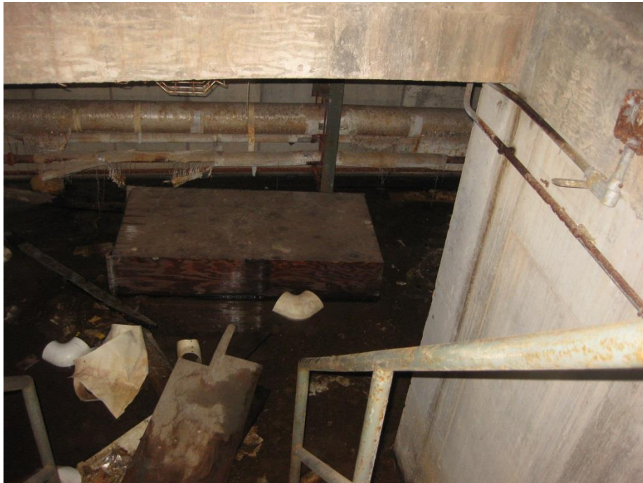
Photo I-4 – Standing Water at Pipe Tunnel
