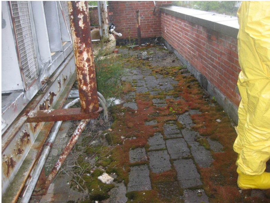
Photo I-2 – Roofing Failure at Boiler Plant
