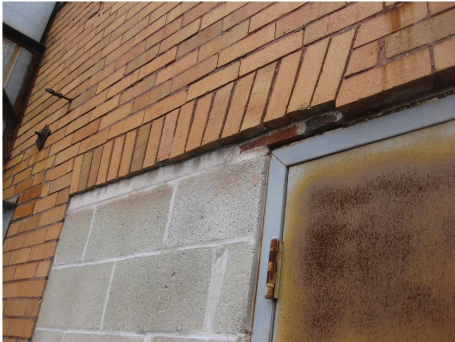
Photo I-6 – Bowed Masonry at Modified Door Opening
