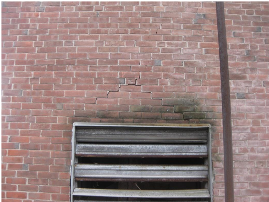
Photo I-5 – Failed Masonry at Vent Opening
