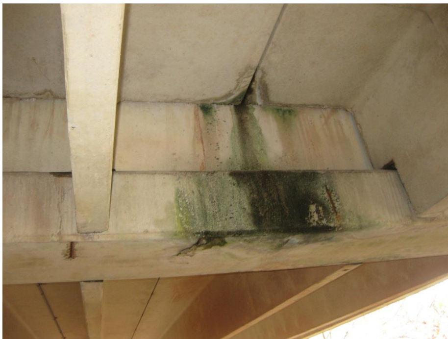
Photo K-4 – Failed Joints Between Precast Elements
