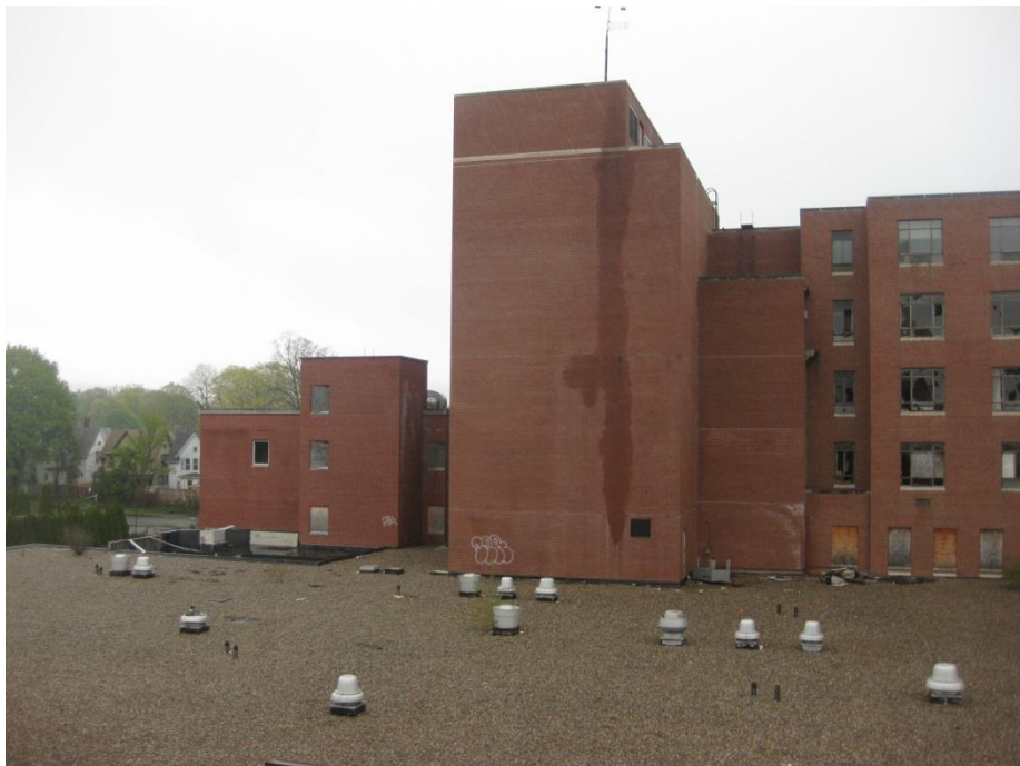
Photo J-1 – Water Infiltration and Rust Jacking at Stair Tower
