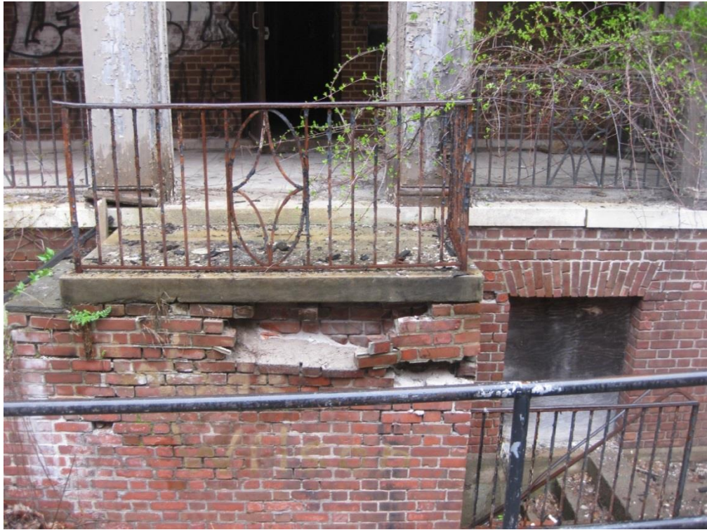
Photo A-3 – Damaged Brick at Wood Structure at Nurses Home
