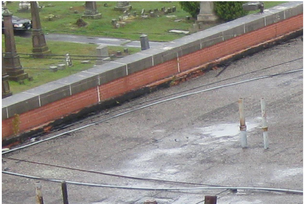
Photo B-2 – Failed flashing at 1966 Addition
