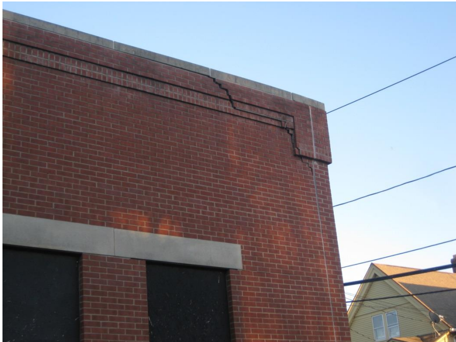
Photo H-1 – Cracked Brick at Corner of Laundry/Storage Addition
