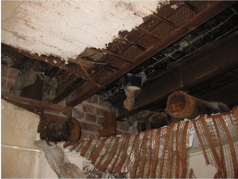
Photo A-1 - Junior Beams and Steel-Tex Floor Slab at Nurses Home
