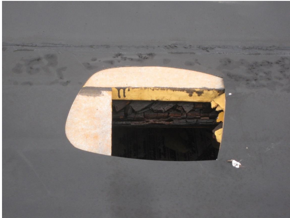
Photo A-5 – Fire Damage at Roof of Nurses Home
