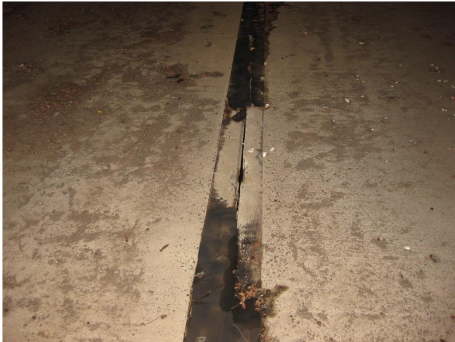
Photo K-7 – Failed Expansion Joint
